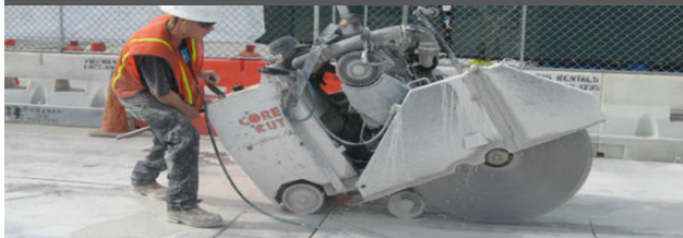
Wet saw cutting. Photo credit: seekkr.com
