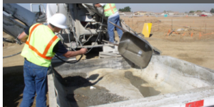
Roll-off system for concrete washout.
